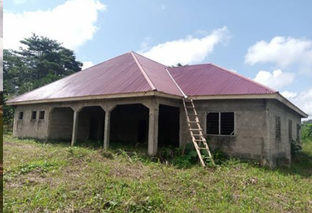
Const. of 1no. CHP Compound at Achiano W.I.P
