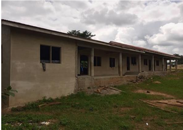
Const. of 3-units JHS classroom blk at W.I.P Dwendaama
