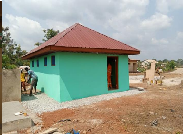
Const. 4 no. WC Toilet Facility at Odumasi
