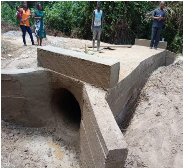
Const. of Pipe Culvert at Endwa-Dwenakyi
